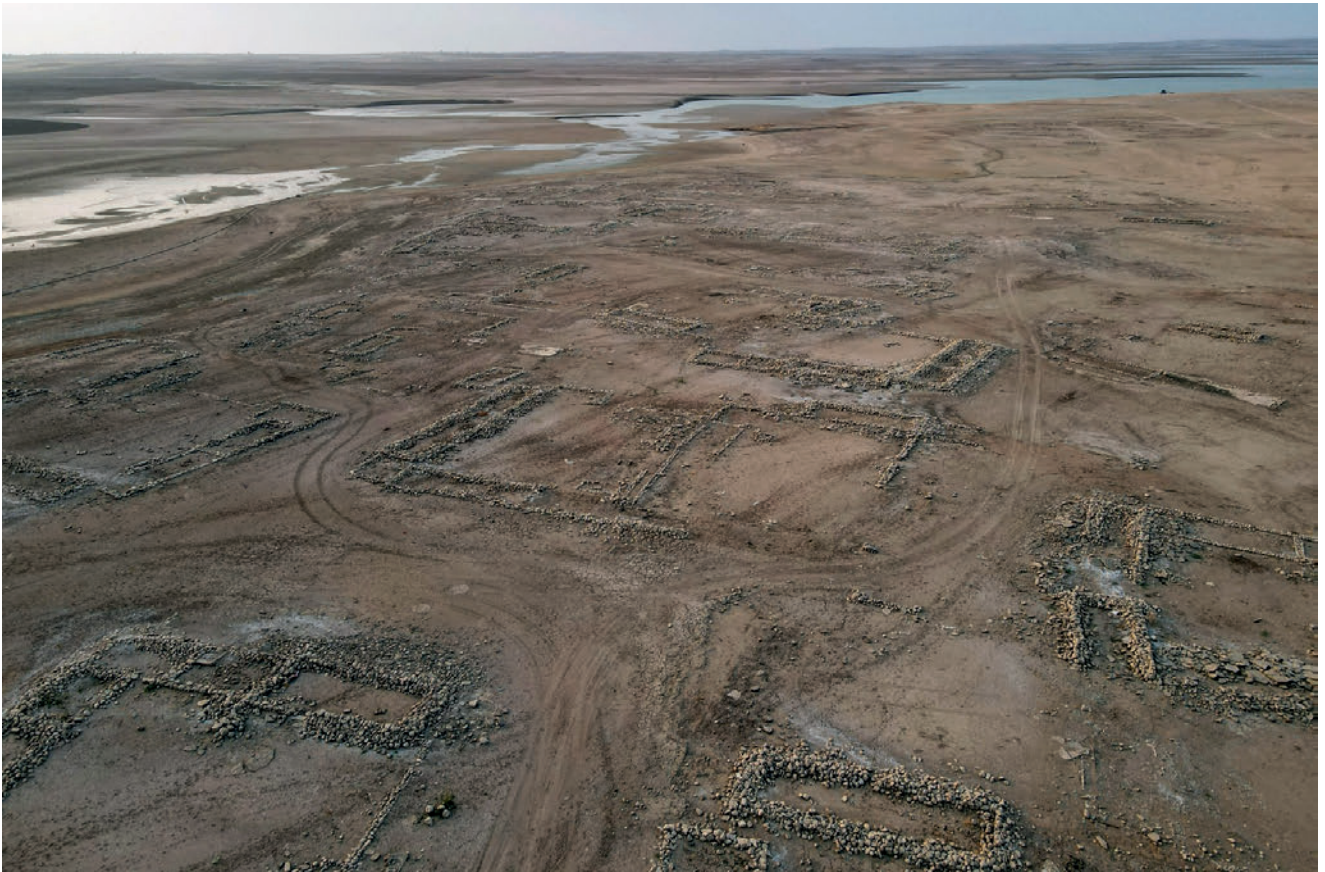
Fig. 8 - The resurfaced village of Anzeh/ReL43 in October 2023 (©ReLand, Photo F. Simi).
