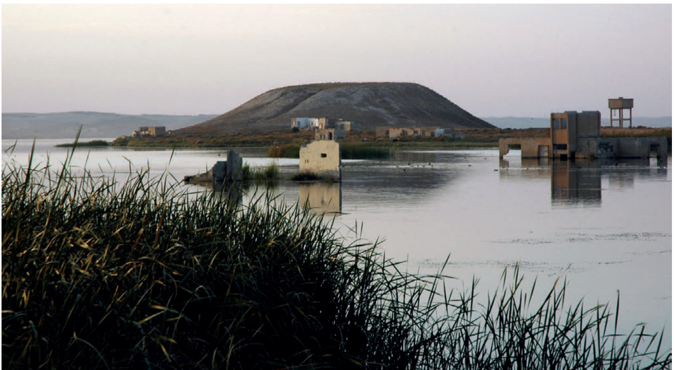
Fig. 2 - Resurfacing houses in the area of Tell Qumluq (courtesy of P. Sconzo).
