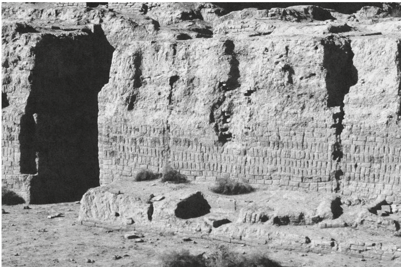
Fig. 4 - The north-west wall of a temple court-yard east of the ziggurat at ‘Aqar qūf. The depth of deposit above the brick wall of the ancient structure can be seen (photograph Tim Clayden, 1985).
